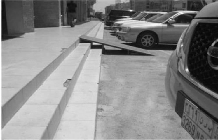
Figure 2. Photo of Iron sheet used as a ramp in a hospital in Amman.
